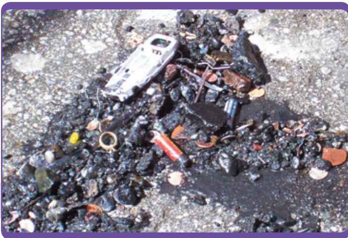
Image #9 – Debris removed from a sewer pipe
