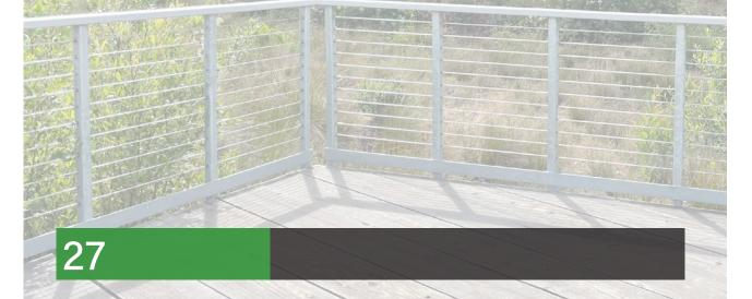
Guardrail with metal posts, wire cables, and a wood cap
