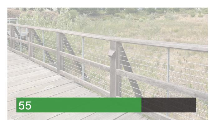
Example of a wooden guardrail with cable wire fencing
