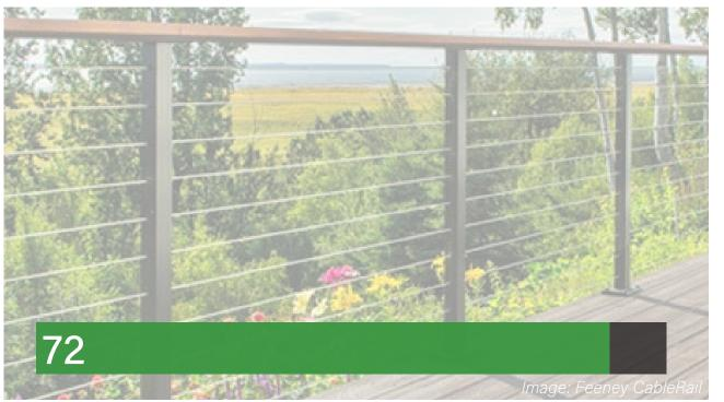
Example of a guardrail with black metal posts, wire fencing, and a wood cap
