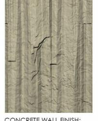
CONCRETE WALL FINISH: BASALT LINER STAINED
