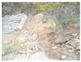
There is a stream coming out at the base of the slope below the distressed portion of Ocean Blvd. On the east side of the road above, there is evidence of uncontrolled drainage coming through the vacant lot. This water may be a contributing factor in the recent movement.
