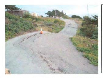
This picture shows Ocean Blvd. from La Grande looking south to San Lucas (see barrier in distance). The road is offset along the cracks by as much as 6" vertically. The angle of dip on the road is from 2 to 20 degrees west.
