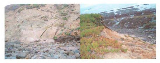
The picture on the left shows part of an old cement "blanket" that sits below the occupied house near the Distillery. It is broken, and the ocean has eroded the rock from behind it. The photo on the right shows the edge (just below the dark green bluff) of another partial blanket of cement that exists downhill of the Ocean Blvd. area that is failing.
