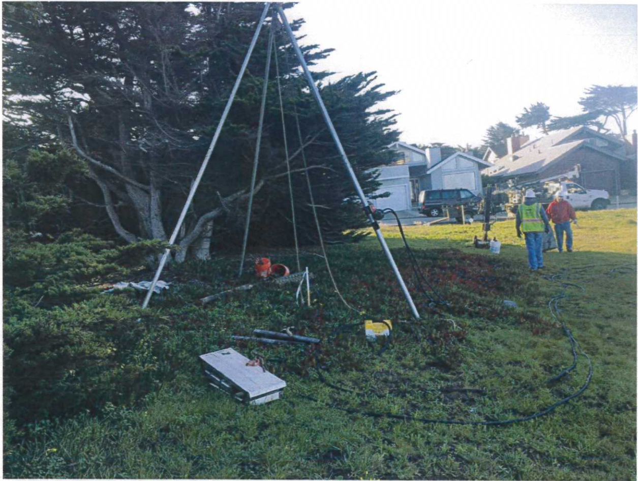
Drill setup test bore hole B4
