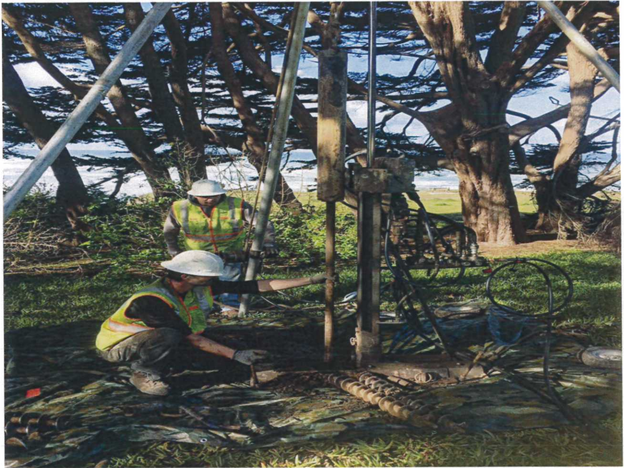
Drilling operations at test bore hole B1
