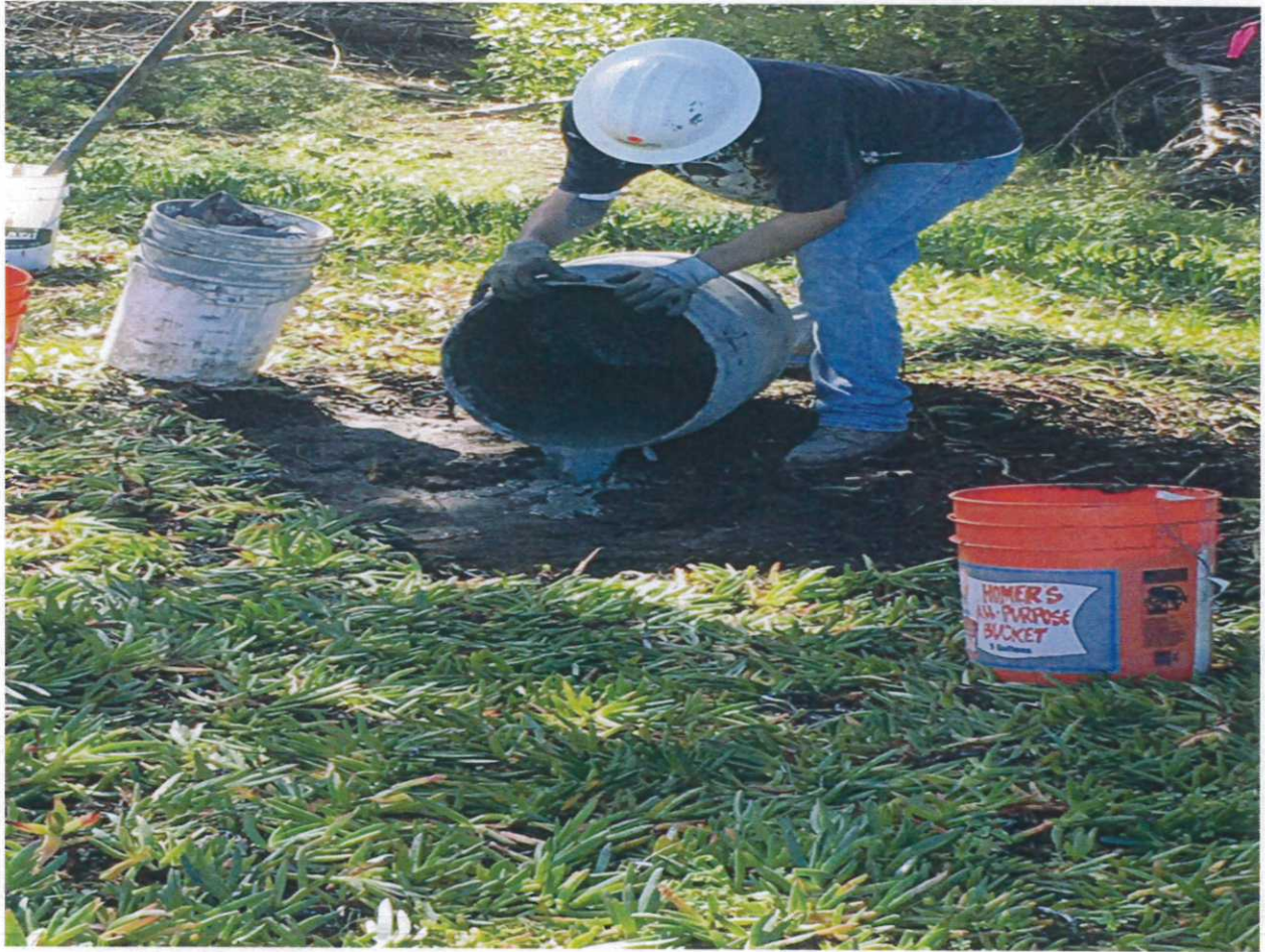
Grouting of test bore hole B1
