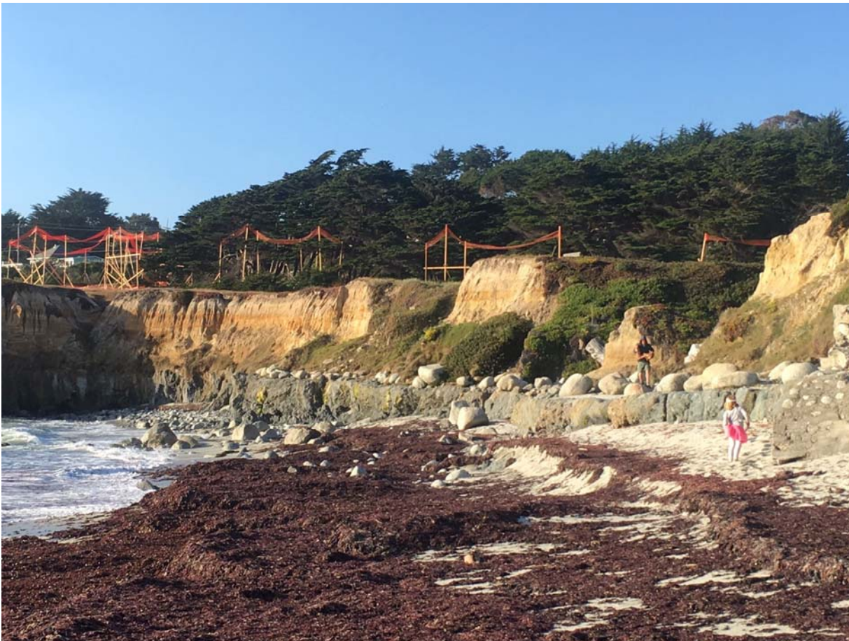
Looking east from Wienke Cove beach. Lot 1 (left) has full story poles; others partial height/number.
