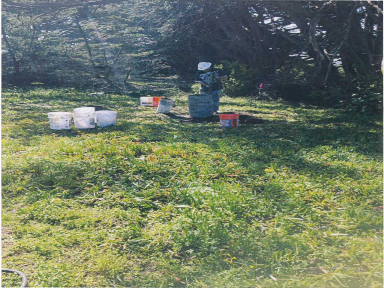
Collection of spoils and mixing of grout at test bore hole B1
