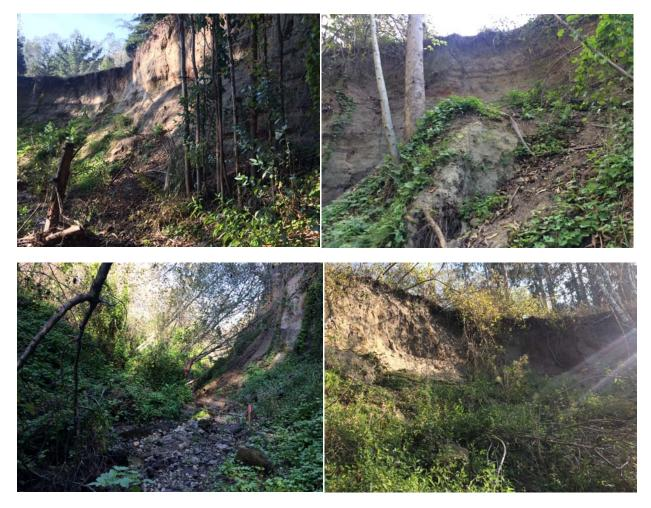
Figure 3 Collapsed Channel near station 0+50, 2+50, 3+50, and 5+00
