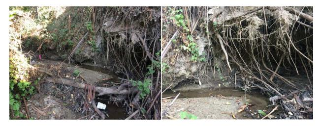
Figure 2 Undercutting near station 1+00
