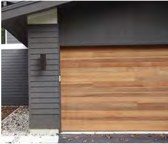
6. GARAGE DOORS: Natural wood Roll up doors - Western Red Cedar - Clr. polyurethane finish
