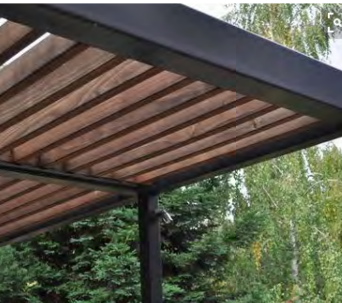
8. OVERHANGS: Natural wood trellis- 4x12 douglas fir beams with clear polyurethane finish
