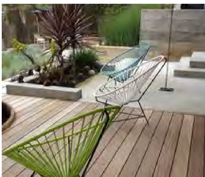
9.HARDSCAPE / DECKS: poured concrete and natural wood decks - 2x6 teak clr. polyurethane finish
