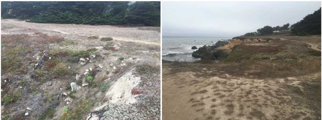
Figure 3 Photos of the bluff top showing concrete debris and fill at the top of an active landslide (left) and the variability in the bluff edge caused by gullies (right)
