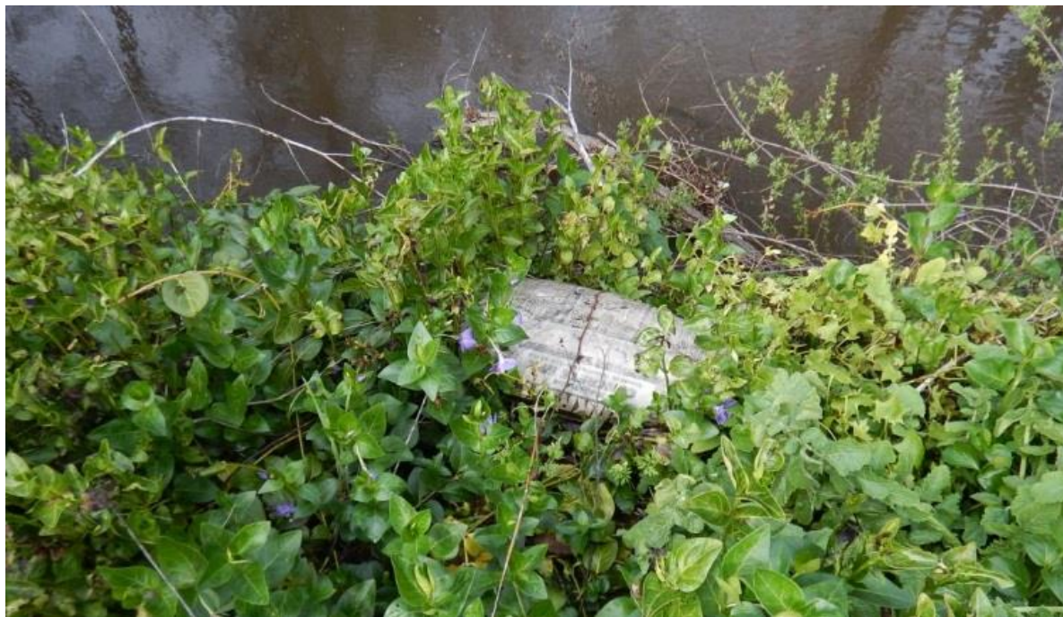
Figure 21. Sackcrete placed below top of bank without permits.
