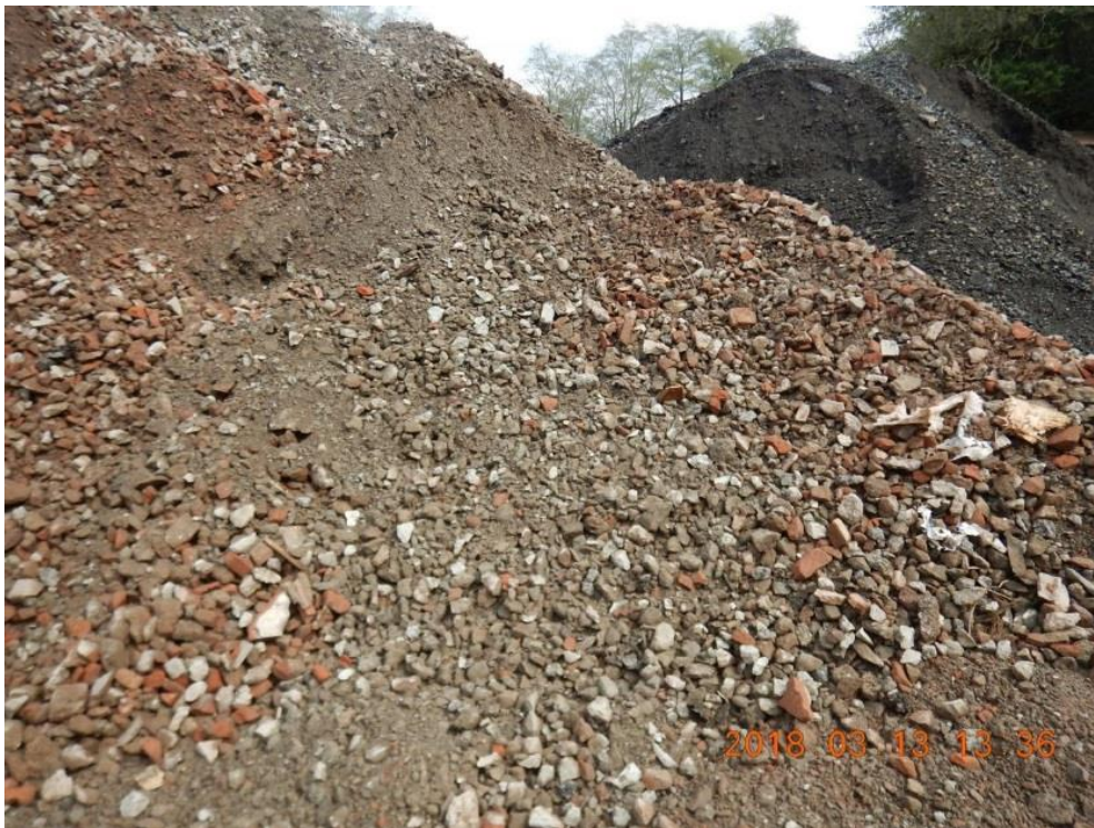
Figure 13. Large pile of construction debris and asphalt in center of flood plain.
