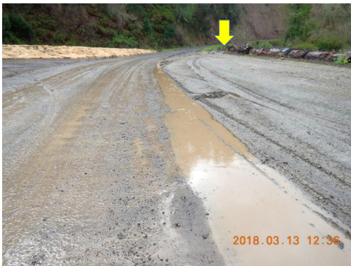
Figure 1. Plume of sediment and contaminant-laden discharge originating on the parking lot area and entering into San Gregorio Creek. Yellow area indicates the point of discharge.
