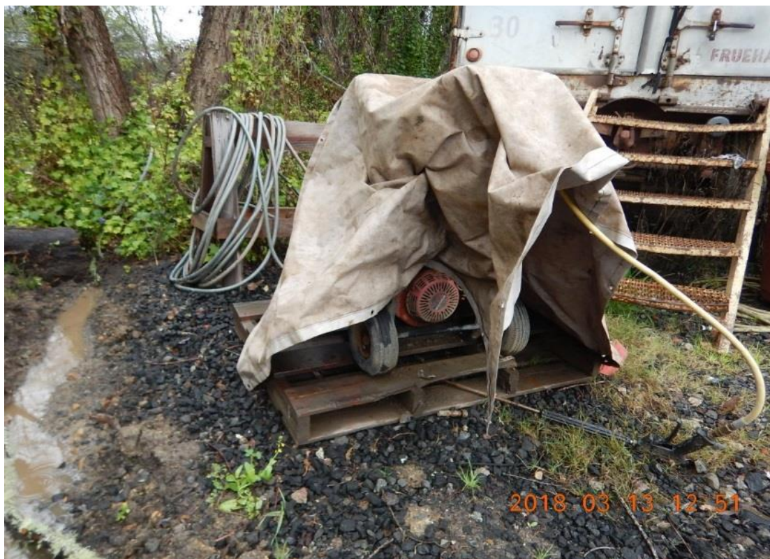
Figure 6. Gas generator (with fuel in the tank) placed at top of left bank with no secondary containment. Sediment laden water is being discharged to San Gregorio Creek immediately to the left in this photo.
