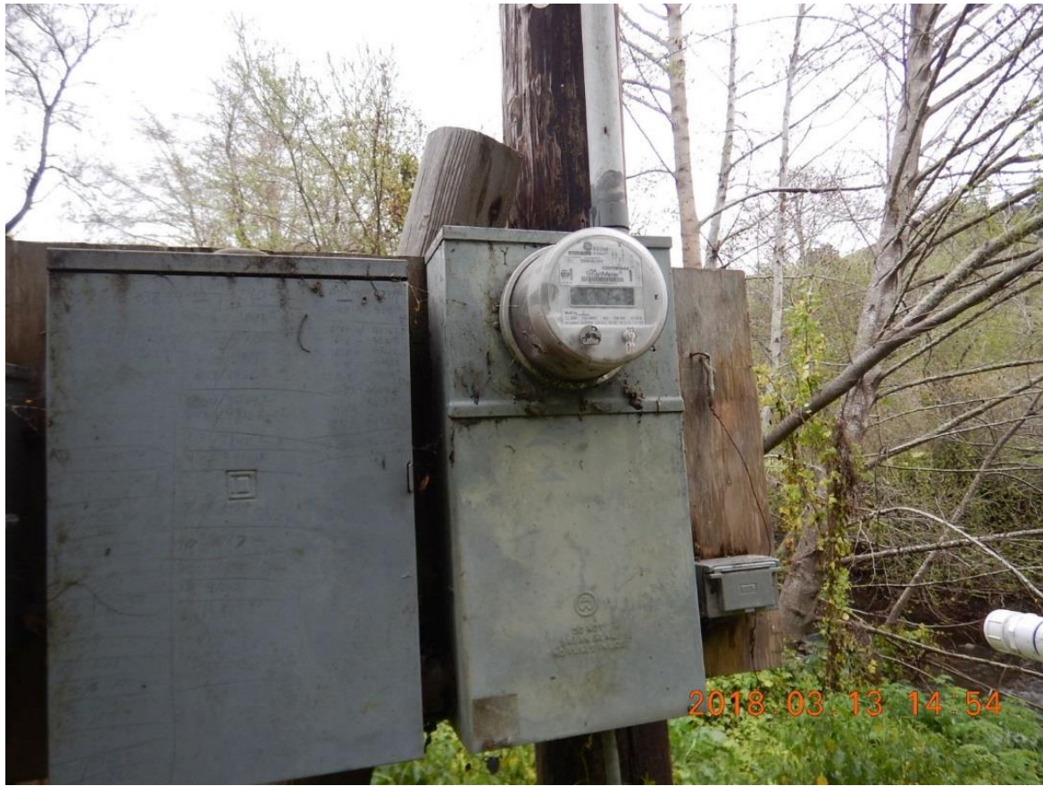
Figure 24. Pump apparatus associated with Point of Diversion #3.
