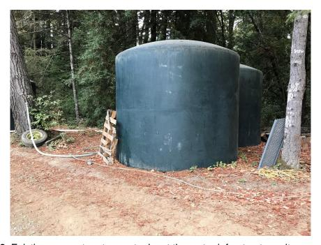
Photo 2. Existing raw water storage tanks at the water infrastructure site.
