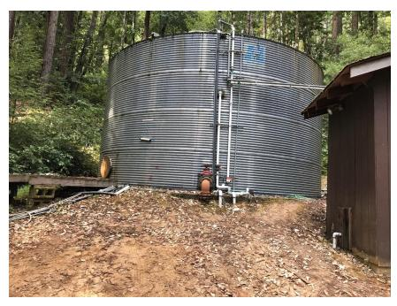
**Photo 3**. The 70,000-gallon raw water storage tank.
