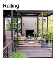
Exotis wood handrail Horizontal cables (4" max. spacing)
