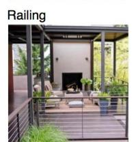
Exotis wood handrail Horizontal cables (4" max. spacing)
