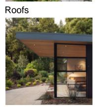
Standing seam zinc clading Grey membrane for flat roof areas
