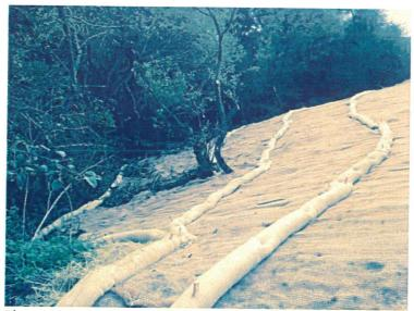
Photo 6: Final erosion control
