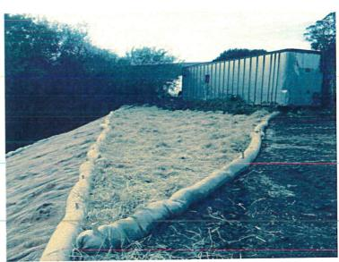
Photo 7: Final erosion control
