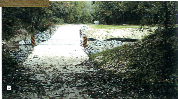
Figure 10. Example of a Vented Ford with Multiple Box Culverts and Grates with Debris Lifters. Example taken from the USDA Forest Service's Low-Water Crossings: Geomorphic, Biological, and Engineering Design Considerations, Appendix A, Case Study 19.
