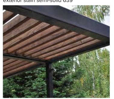
8. OVERHANGS: Natural wood trellis-4x12 douglas fir beams with clear polyurethane
