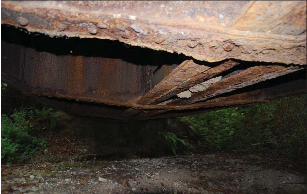
Figure 6: Harkins Bridge, redundant box girder and stringers
