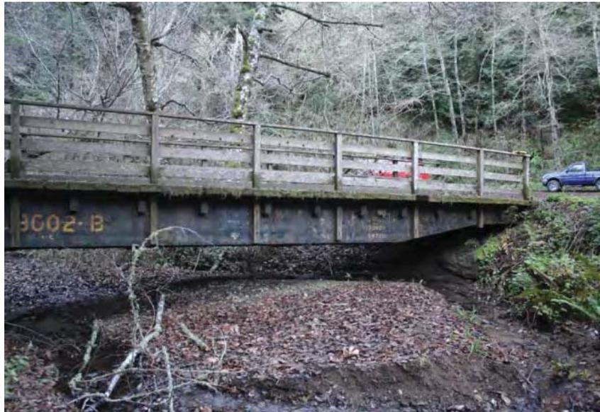
they still have plenty of capacity to support even the heaviest highway trucks, HS20 loading. It is questionable whether or not abutments exist under the girder ends – none were observed. It is possible that the girders are placed directly on soil. Regardless, this system appears to be functioning adequately.
