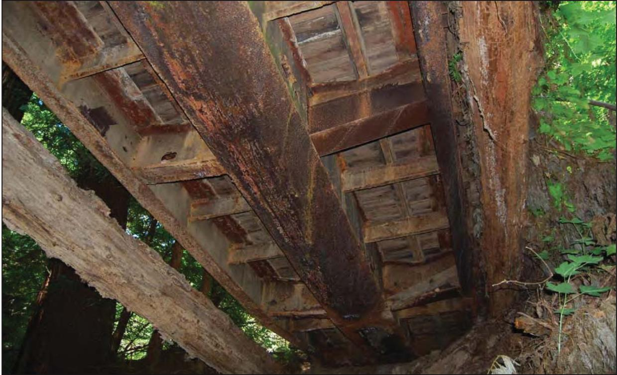
Figure 13: Soda Gulch Bridge, non-redundant main box girder with stringers, exterior girder and floor beams
