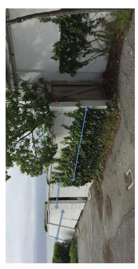
South fence section and double gates proposed for removal have failed and are leaning against the Cypress behind.
