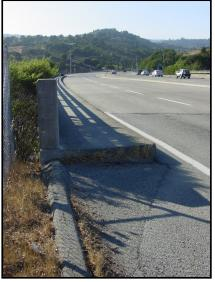
Sidewalk with no curb ramp on SR92 Overpass, between the signalized study intersections
