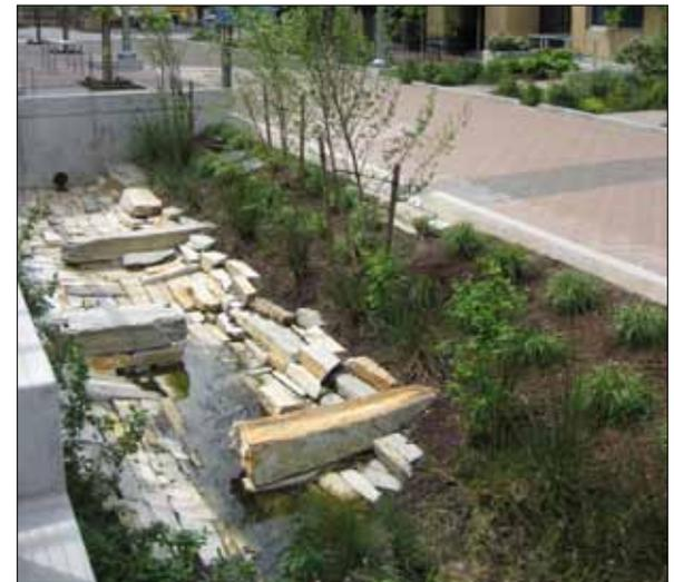
*Creative on-site retention facilities to detain, treat and reuse stormwater for irrigation are required for new development*
