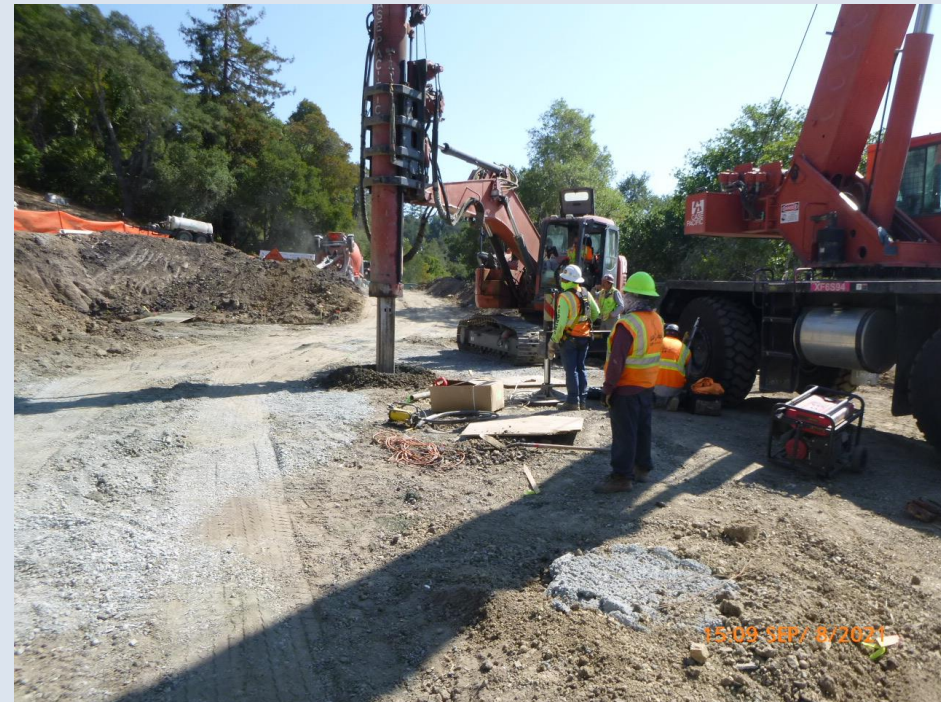
Drilling of piers for retaining wall
