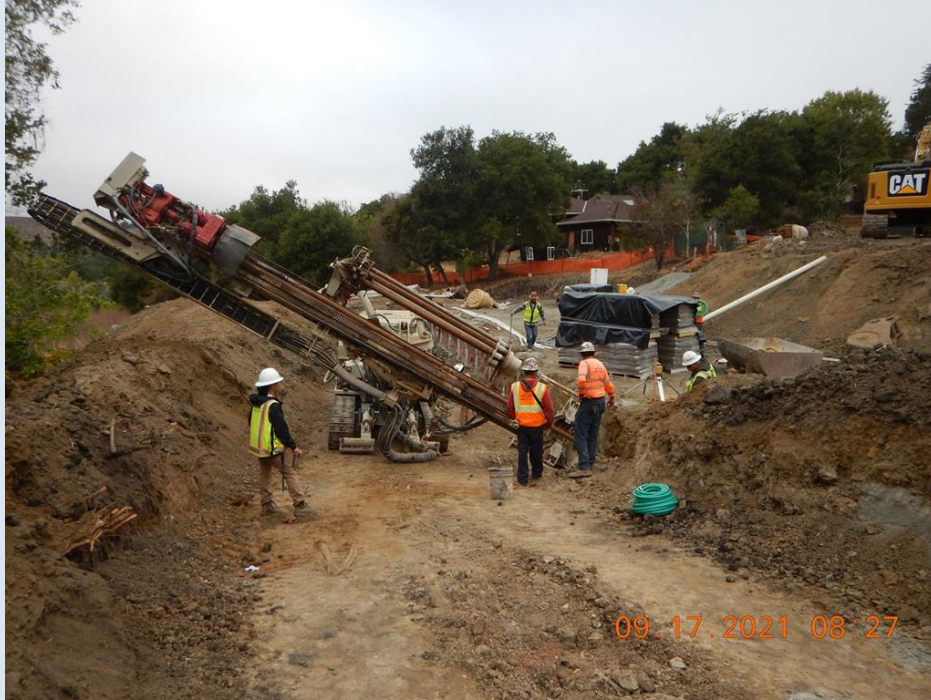
Drilling of tie-back anchors for retaining wall
