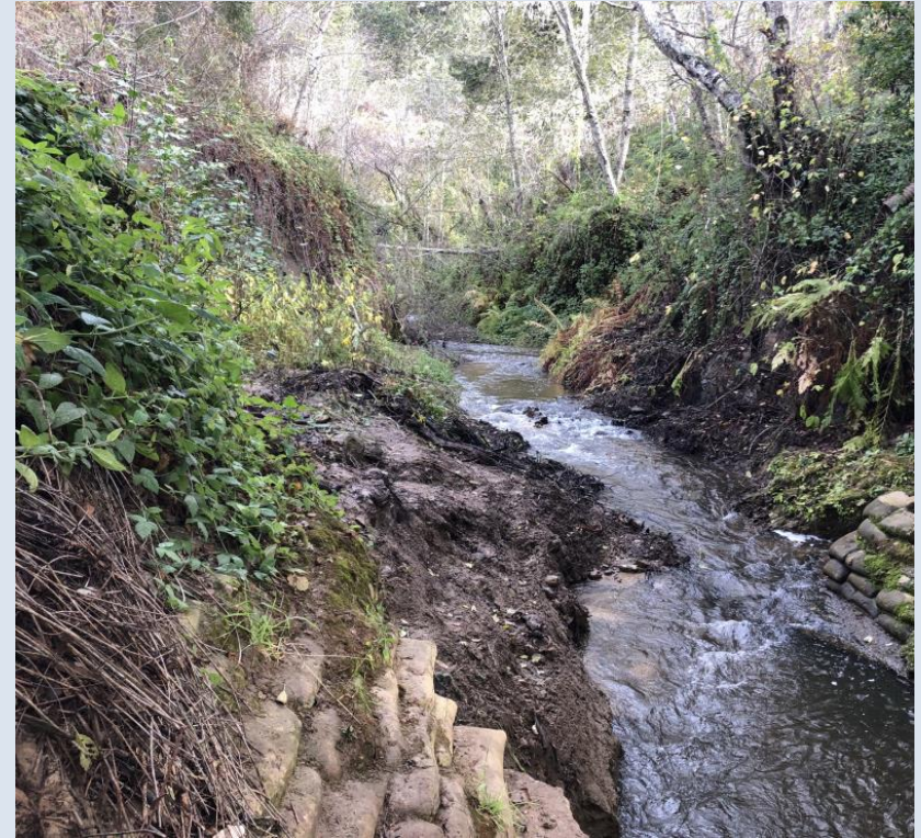
Butano Creek Pre-Construction – Concrete Sack Bank Protection
