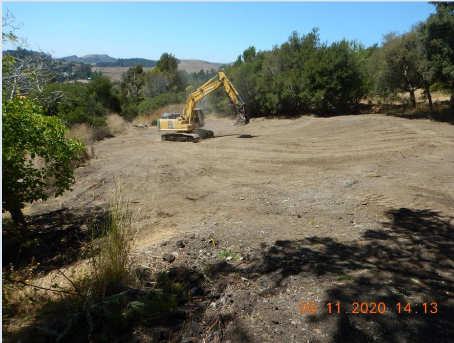
Final grading for where home was demolished
