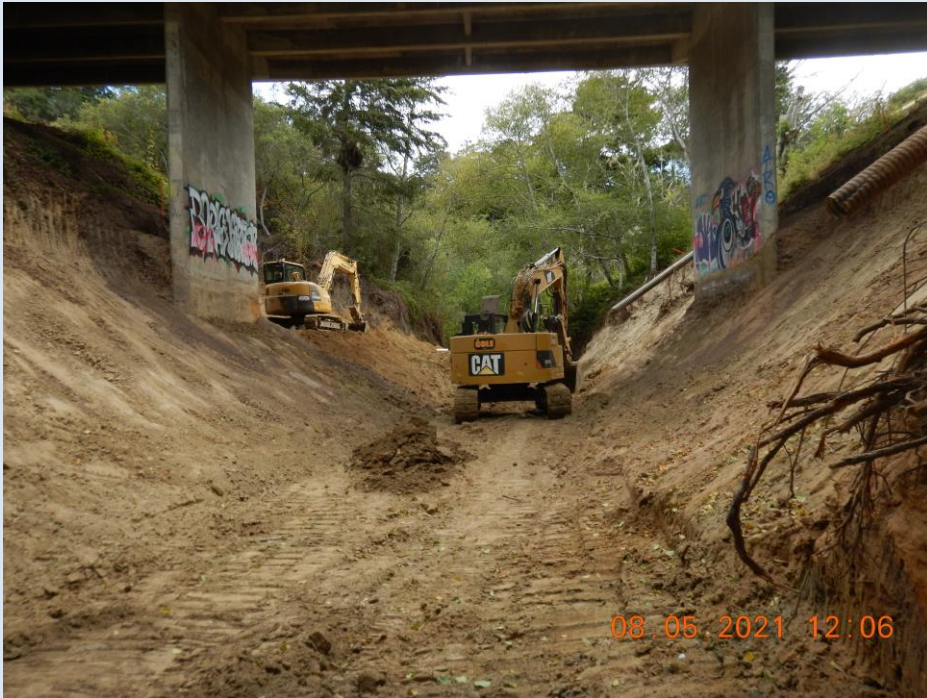
Grading underneath in preparation of rock placement
