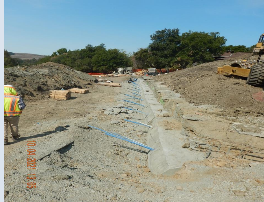
Concrete waller completed with tie-backs
