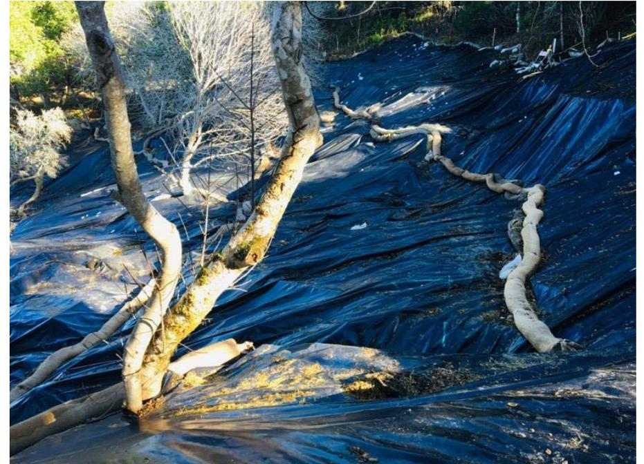
District maintenance staff continue to operate & monitor the temporary pump bypass system at the mudslide site in the easement behind Seneca Lane; Maintained winterization measures prior to the 2018-19 rainy season to minimize further erosion; Working with consultant and FEMA to finalize design of permanent repair.
