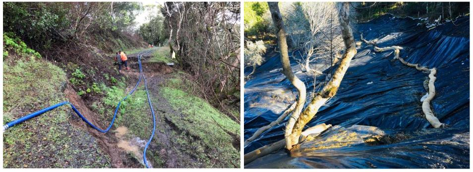
District maintenance staff continue to operate & monitor the temporary pump bypass system at the mudslide site in the easement behind Seneca Lane; Maintained winterization measures prior to the 2018-19 rainy season to minimize further erosion; Working with consultant and FEMA to finalize design of permanent repair.
