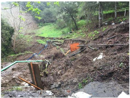
Jan. 24, 2017 – Feb. 15, 2017: District maintenance staff responded to a mudslide that damaged a section of the District's sewer main in the easement behind Seneca Lane, installed temporary bypass system, and monitored the bypass pump system 24 hours/day until PG&E approved a power connection.
