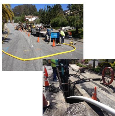
Replaced 2,230 feet of pipes in easements & 8,540 feet of pipes in streets (11% of District mains) funded by State Revolving Fund Loan with 20-year term and interest rate @ 2.1%
