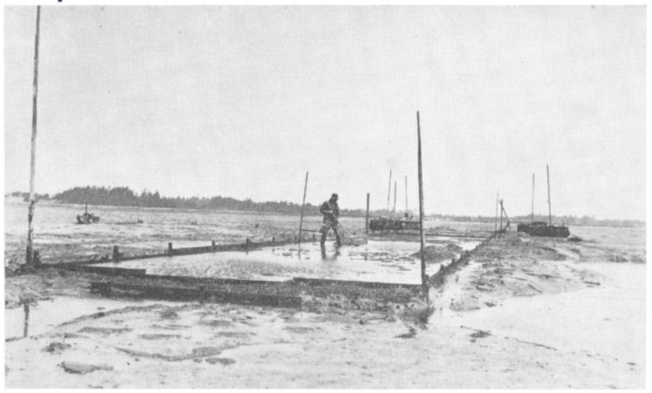
FIGURE 30. Diked, gravelled bed under construction, south San Francisco Bay, 1933.
