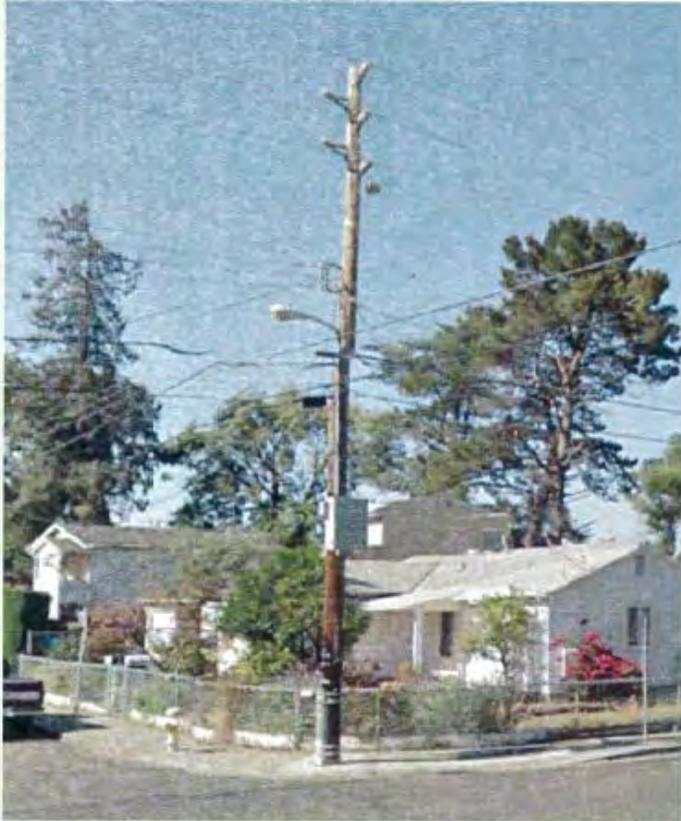
Alternate Pole East #2- Structurally the pole would have to be replaced to place equipment on pole.
