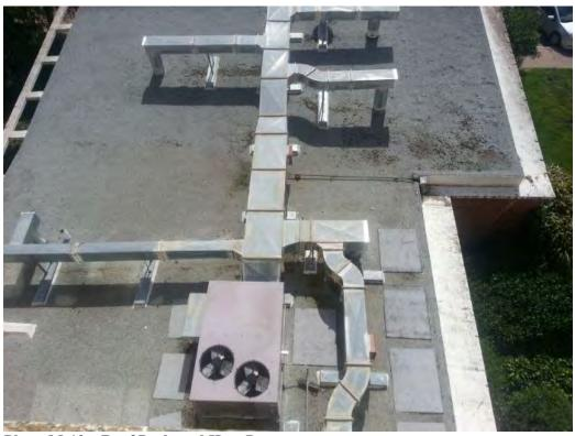
Photo M-10 - Roof Packaged Heat Pumps
