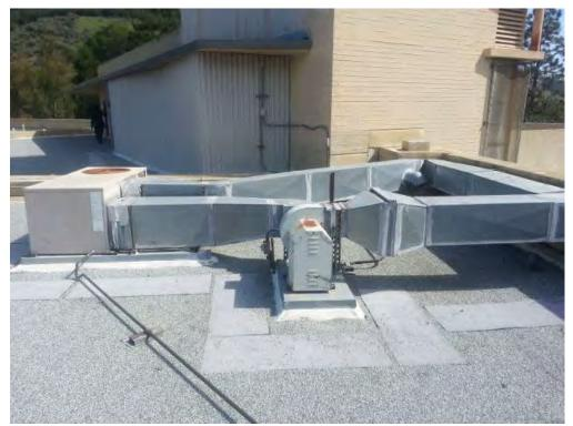
Photo M-9 – Roof Packaged Heat Pumps
