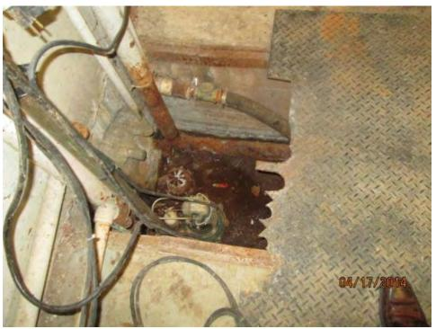
**Photo P-5 - Sump Pumps in Trench**
