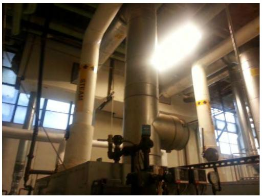
**Photo M-2 – Boiler Flue**
