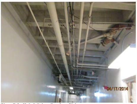
Photo P-2 - Hub & Spigot Cast Iron Piping
