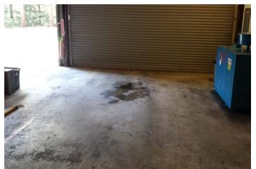
Photo 13: View of minor hydrocarbon staining inside Apparatus Building
