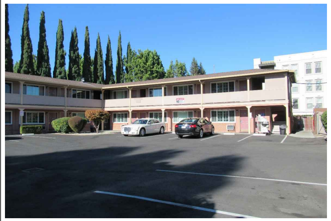
Rooms at Rear of Property
