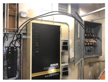
ISD team members crafted a temporary power rewire solution to bypass failed equipment
