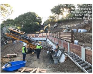
Drilling for placement of the second row of tie-backs in wall
