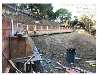
Formwork for waler where the tie-backs will be placed
