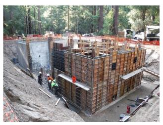
Rebar and formwork for WWTP tank sidewalls
