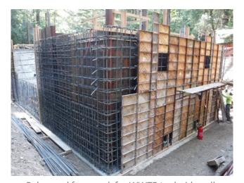
Rebar and formwork for WWTP tank sidewalls
