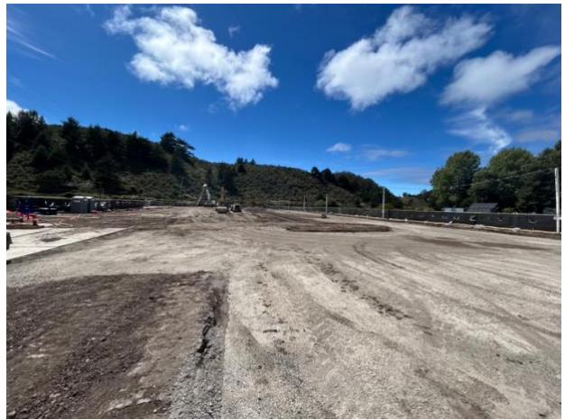
Site Grading in progress
