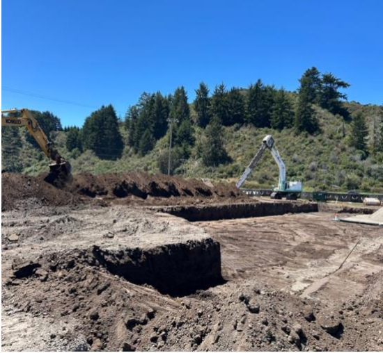
Site grading in progress
