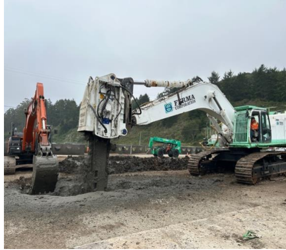
Ground improvements in progress
