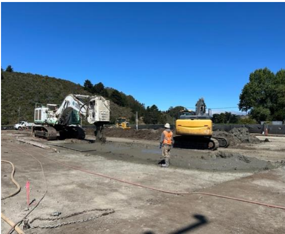
Ground improvements in progress
