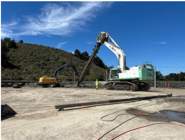
Ground improvements in progress
