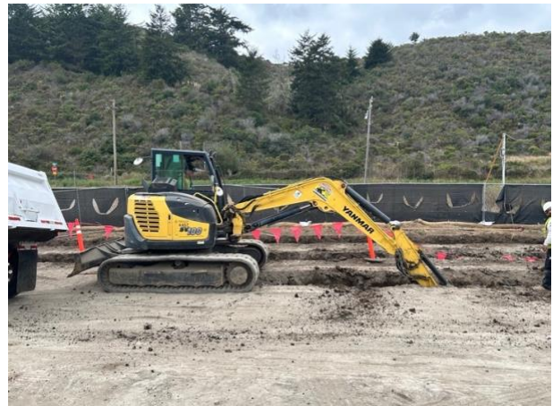
Ground improvements in progress
