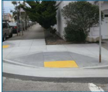
New Accessible Curb Ramps
