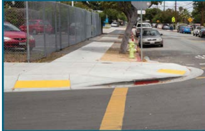
New Accessible Curb Ramps
