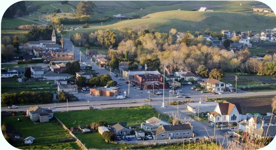
Pescadero microgrid project
