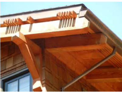
Building with copper flashing, gutter and drainpipe.
