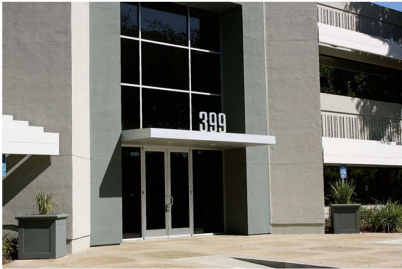
Canopy at Entrance
