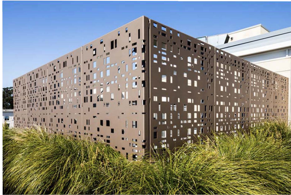
Mechanical Roof Screens
