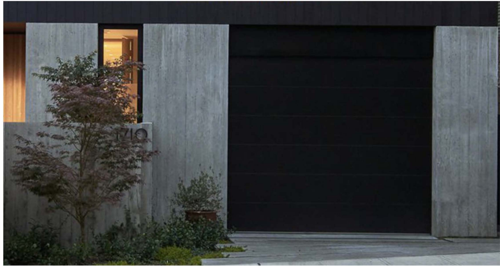
Concrete Wall Exterior Vertical Formed
