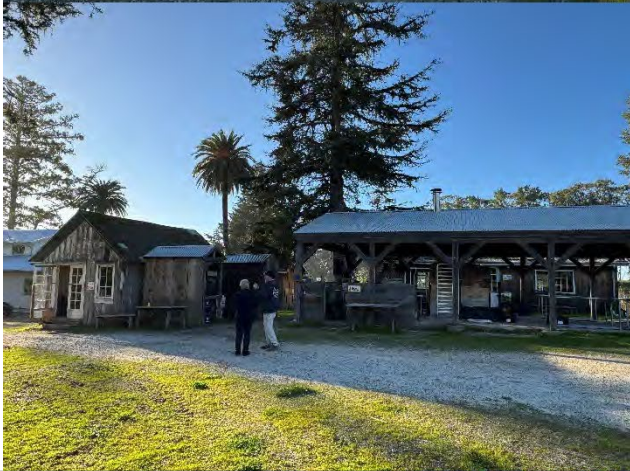
East side of outdoor kitchen and shed
