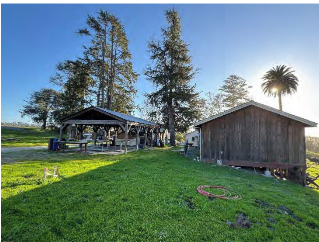
North ends of kitchen and classroom
