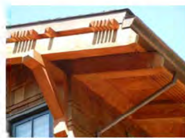
Building with copper flashing, gutter and drainpipe.
