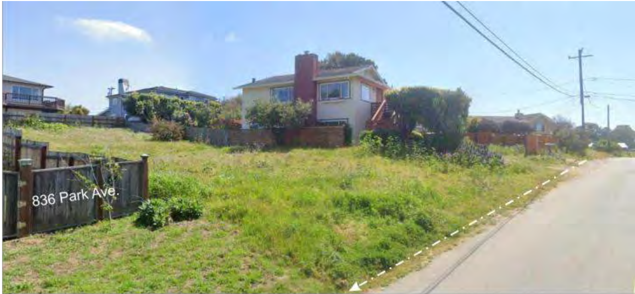
Northeast Google Earth Pro street view across gentle southwest sloping, grass-covered parcel. Note good condition of San Ramon Avenue AC pavement. Northeast side of crowned San Ramon Avenue drains in earthen ditch northwesterly from divide in distance across parcel frontage (white dash-dot line).
