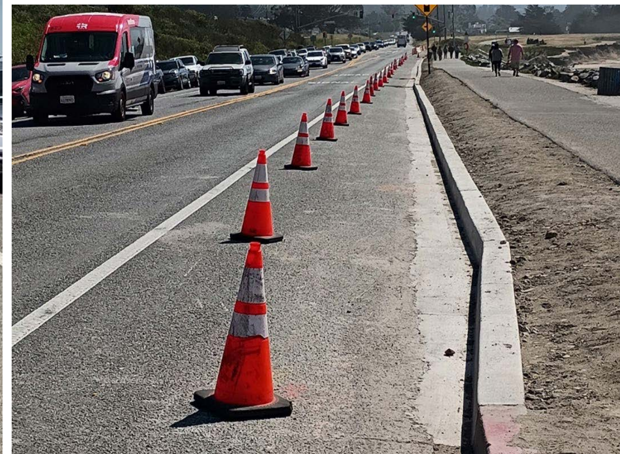
Hwy 1 - Curb Construction on the Westside Near Project Site
