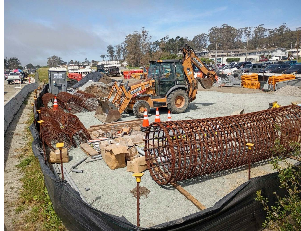
Caltrans portion of Dirt Lot Used for Construction Storage
