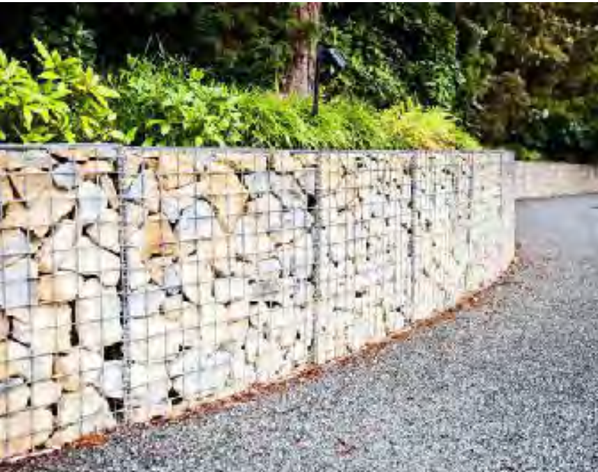
TYPICAL GABION WALLS & GABION BENCHES
