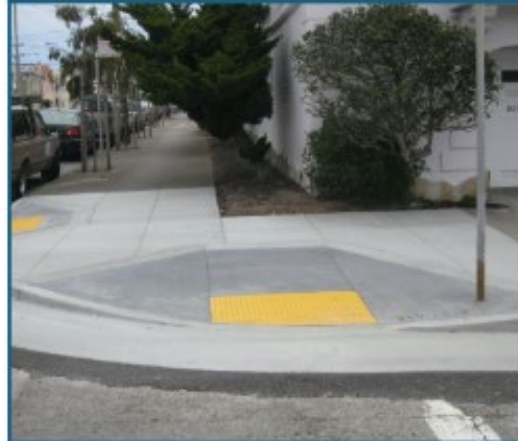
New Accessible Curb Ramps
