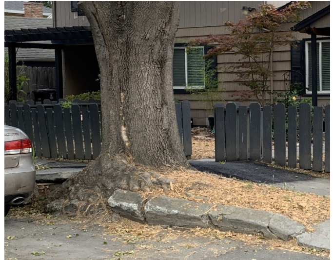
Tree roots uplifted sidewalk and curb. Drainage is affected and ponding could occur.
