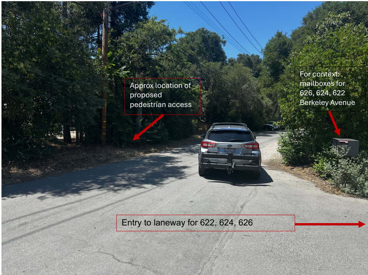
Photo taken on Berkeley Avenue in front of entry to laneway serving 622, 624, 626 Berkeley Avenue, looking toward Colby Ave and Bay Road. Note narrow roadway with limited shoulders (PGE pole on the left side, vegetation on the right side) and limited line of sight to oncoming traffic. There is insufficient space for a car to pass in the opposite direction and insufficient space to pull onto shoulder.
