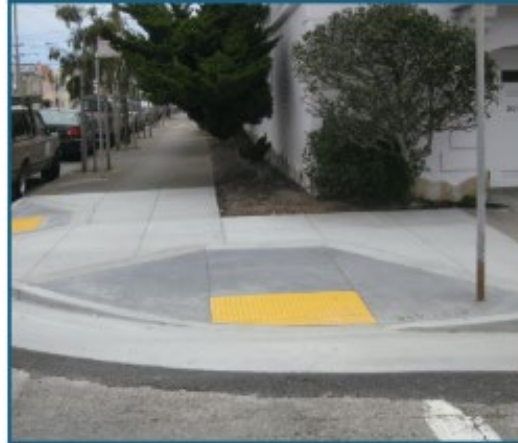
New Accessible Curb Ramps
