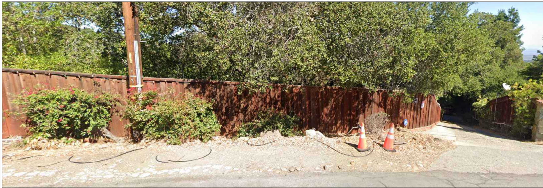
3 EXISTING FENCE PHOTO A0.4 NTS
