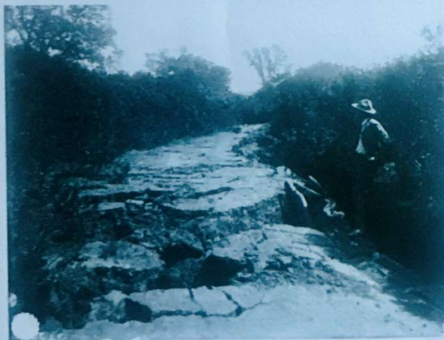
Alpine Road shortly after the M7.9 1906 earthquake. Vertical offset of Alpine Road 5 miles west of Stanford University. Per J. C. Branner. The wide rift in the foreground was created by the rupture of the San Andreas fault but crosses the 1906 fault trace at an angle. This 1906 photograph was published in The California Earthquake of April 18, 1906: Report of the State Earthquake Investigation Commission (1908) . Digital copy from the Andrew C. Lawson Collection, BANC PIC 1957.007, The Bancroft Library, University of California, Berkeley. Courtesy of UC Berkeley, Bancroft Library.
