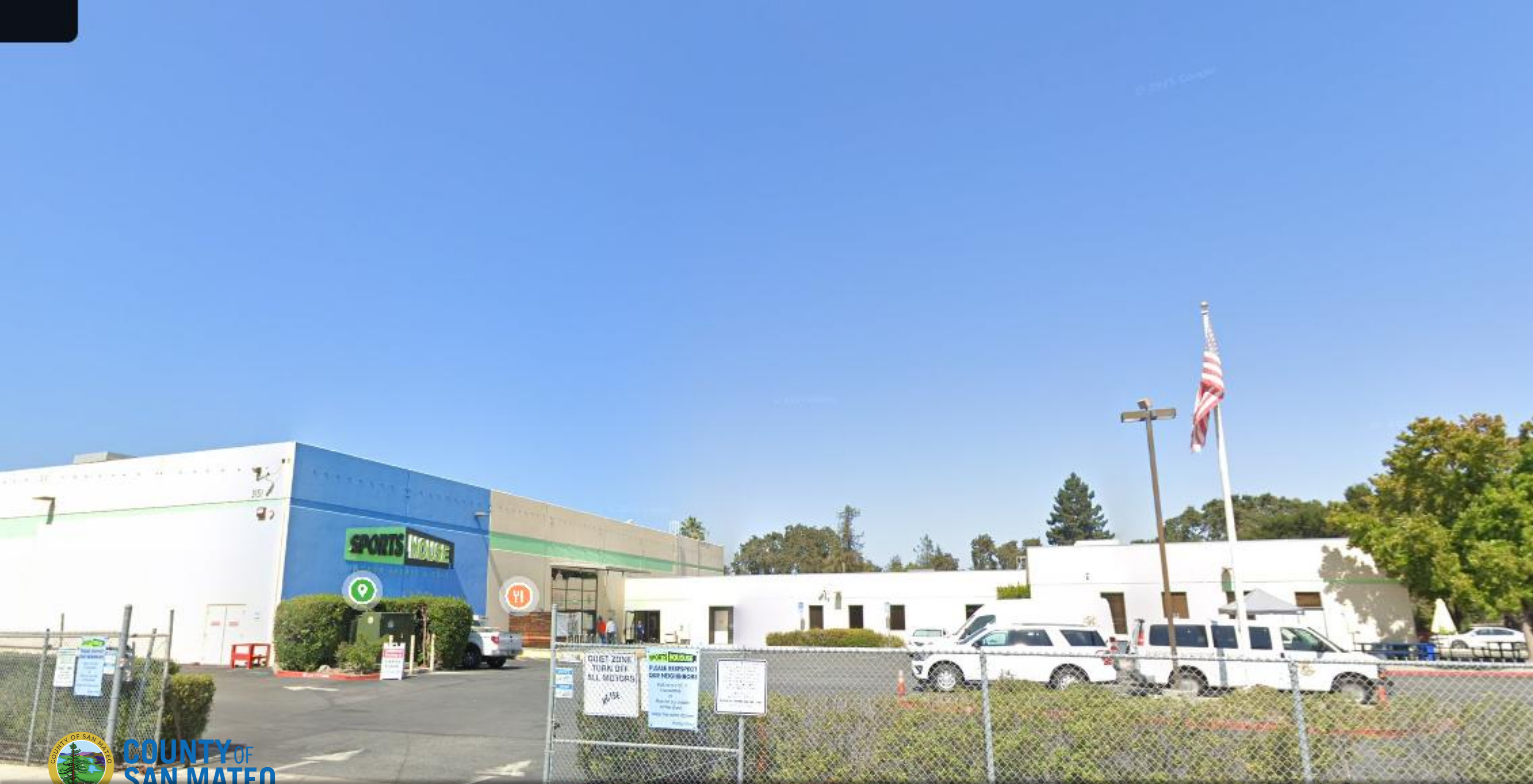
Project will occupy the eastern portion of the building
