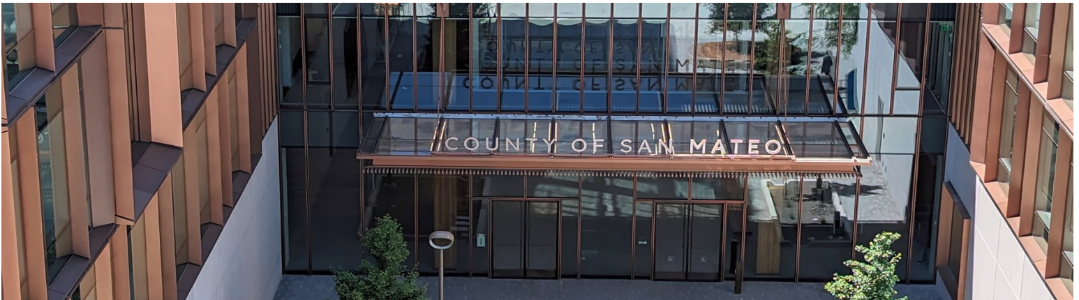
County Office Building 3, Redwood City @ County of San Mateo
