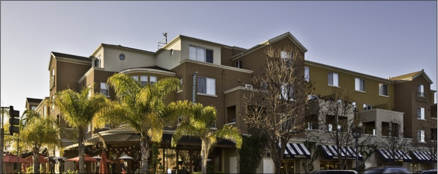
City Center Plaza—Redwood City @ County of San Mateo
