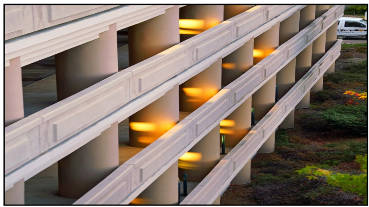
Public Parking Garage at Dusk - County Center @ County of San Mateo
