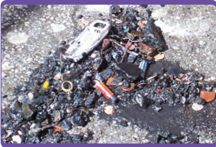
Image #9 – Debris removed from a sewer pipe
