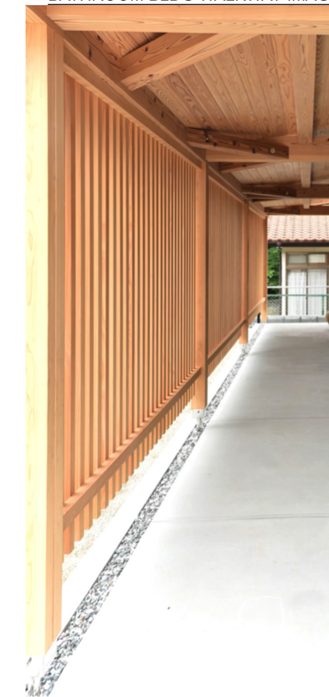
BATHROOM BLDG WALKWAY IMAGE
