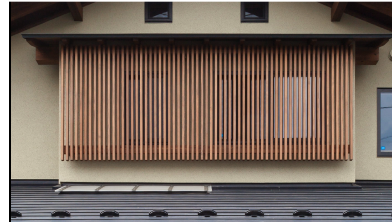
SLATTED WOOD WALL PANEL MATERIAL: RED CEDER
