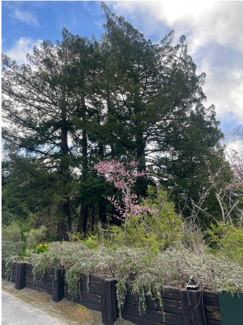
Photo 3 — Looking north-northeast, another view of the retaining wall that will be replaced on the east side of the driveway after it is widened at at 10707 La Honda Road, Woodside, CA 94062 (San Mateo County) (Assessor's Parcel 078-190-210).
