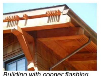
Building with copper flashing, gutter and drainpipe.
