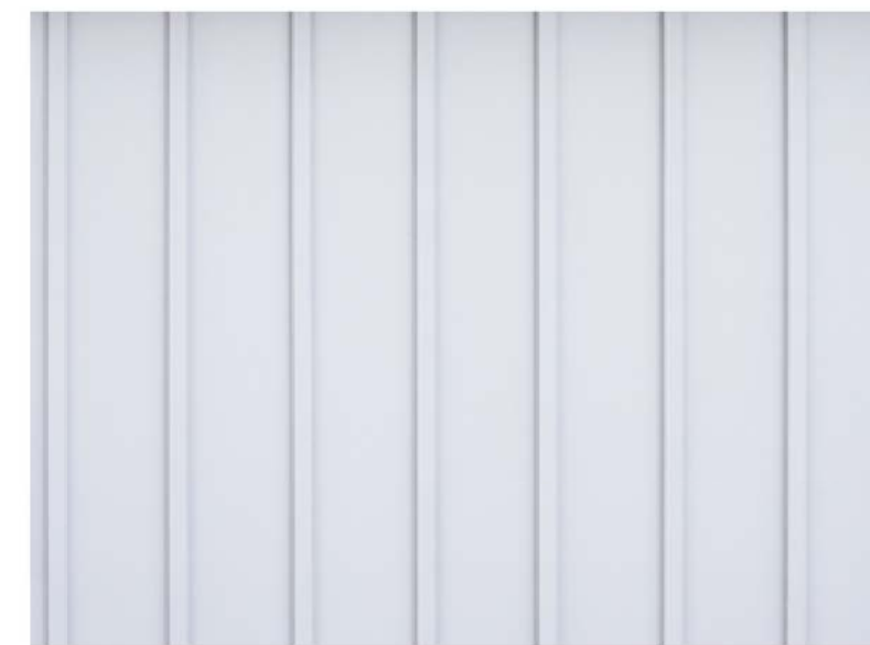
Hardie Panel Board # Batten Siding Painted BJM OC-117 "Simply White"
